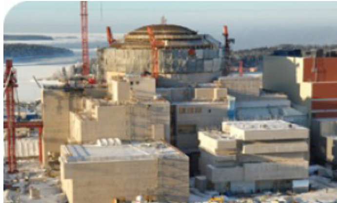
Figure 2.11 Olkiluoto EPR Under Construction
