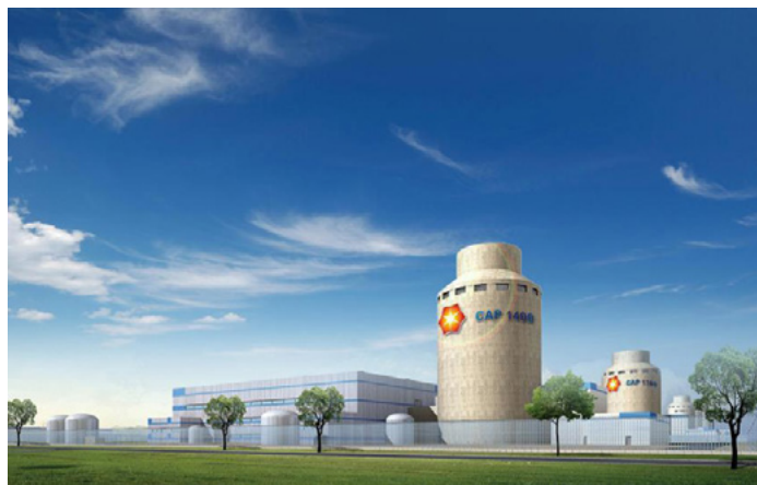
Figure 2.19 CAP-1400 Plant Under Construction in the Shandong Province
