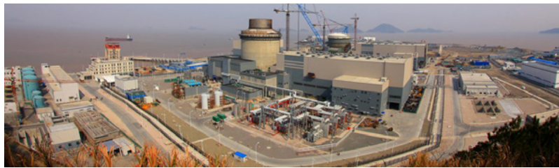
Figure 2.3 Sanmen AP-1000 Under Construction in China
