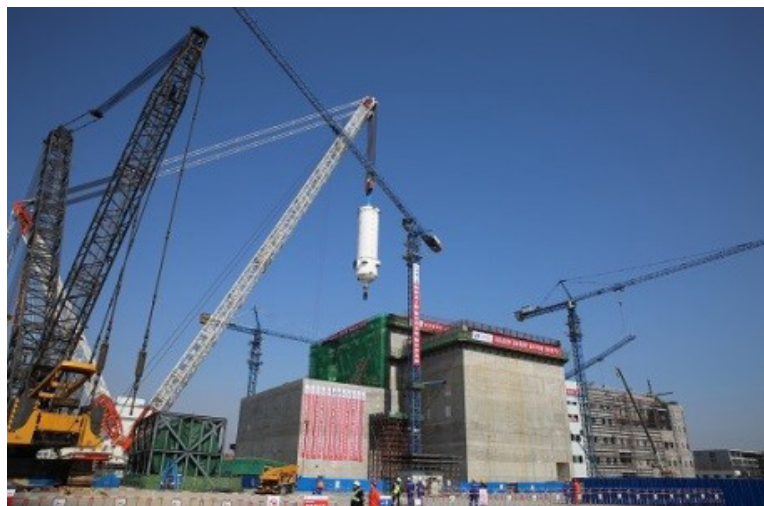
Figure 3.4 HTR-PM Under Construction
